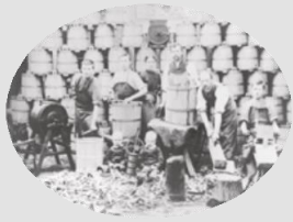
Foundation cooper's workshop Leifeld
